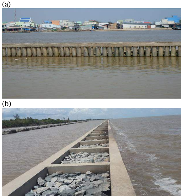
Fig. 1 Double-row pile breakwater
