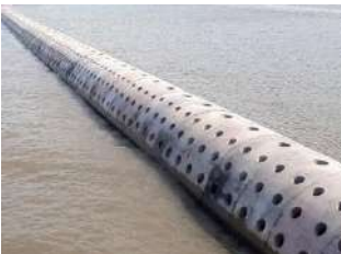
(Hollow circular breakwater)
