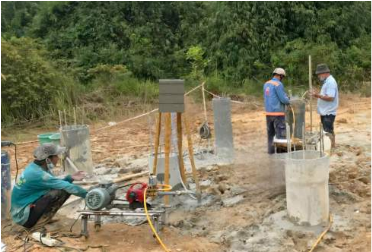
Fig. 9 The grouting process
