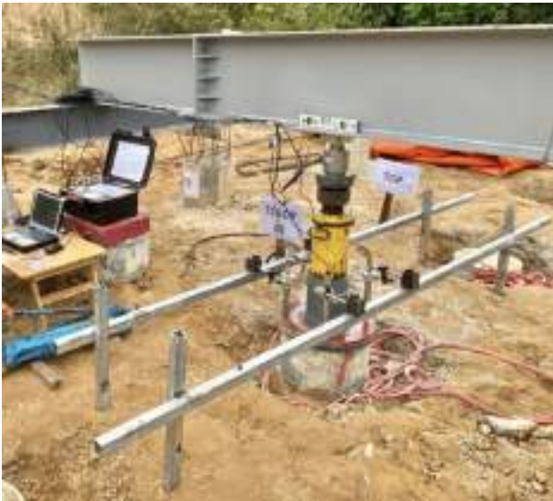
Fig. 10 Instrumentation setup for the field static load test
