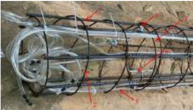
Figure 3.4. Bored-pile reinforcement cage fabricated in the workshop
